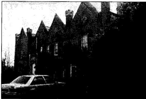
Front of the oldest part of Wallingwells Hall near Worksop. One of many photos taken during Ken and Eve Durnall's visit of 28th April 1989. Photo: Eve Durnall
